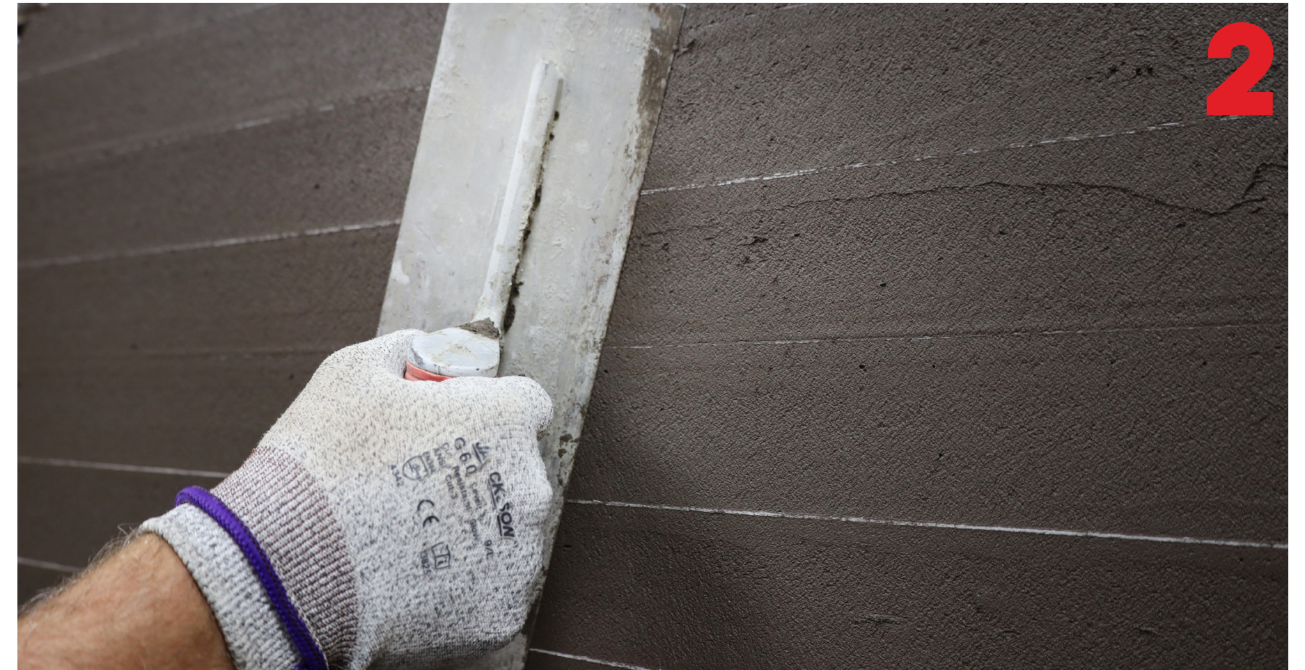
2. Apply mortar to panel.
