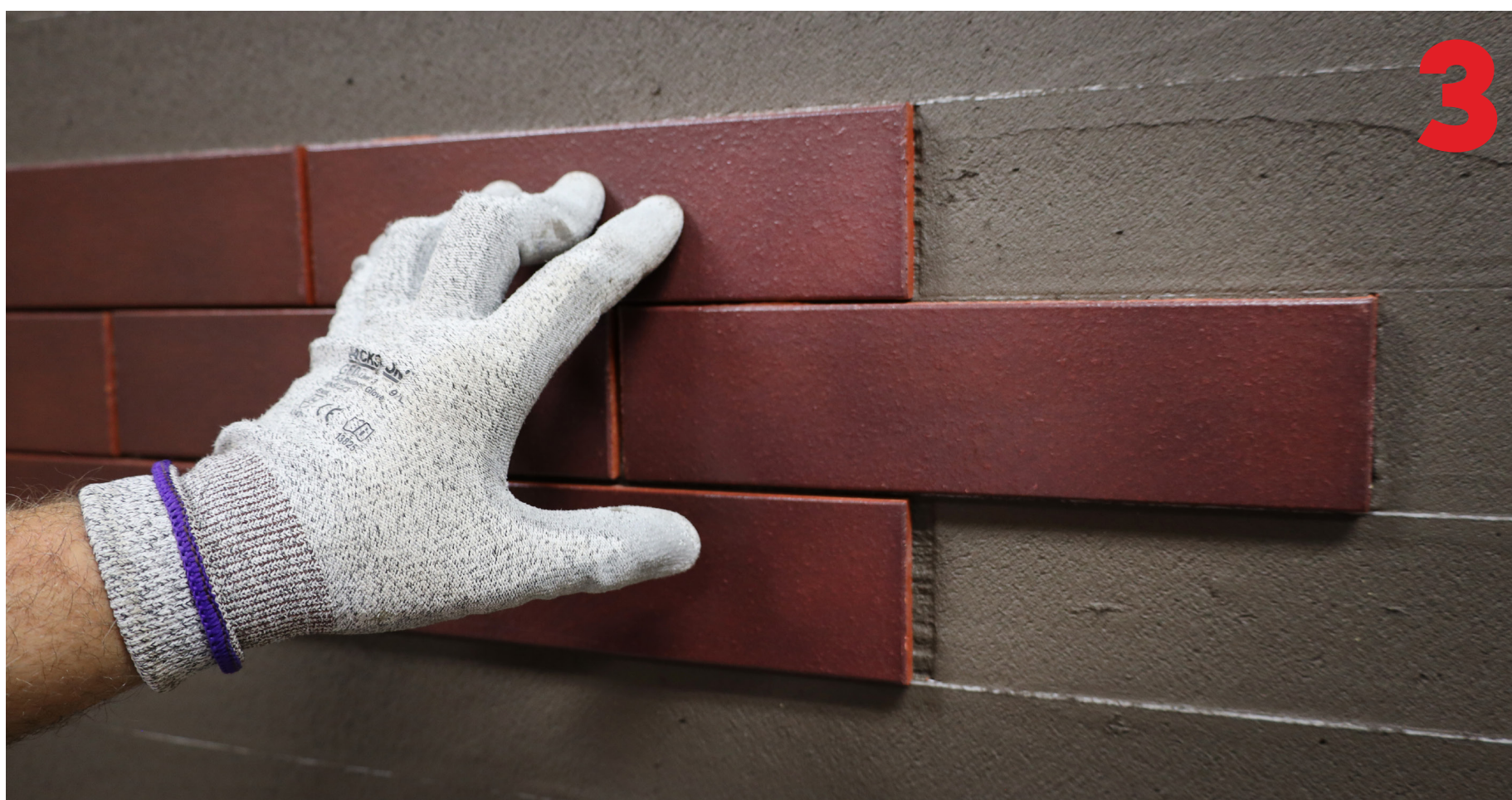
3. Place Ultra-Speed thin brick on panel.
