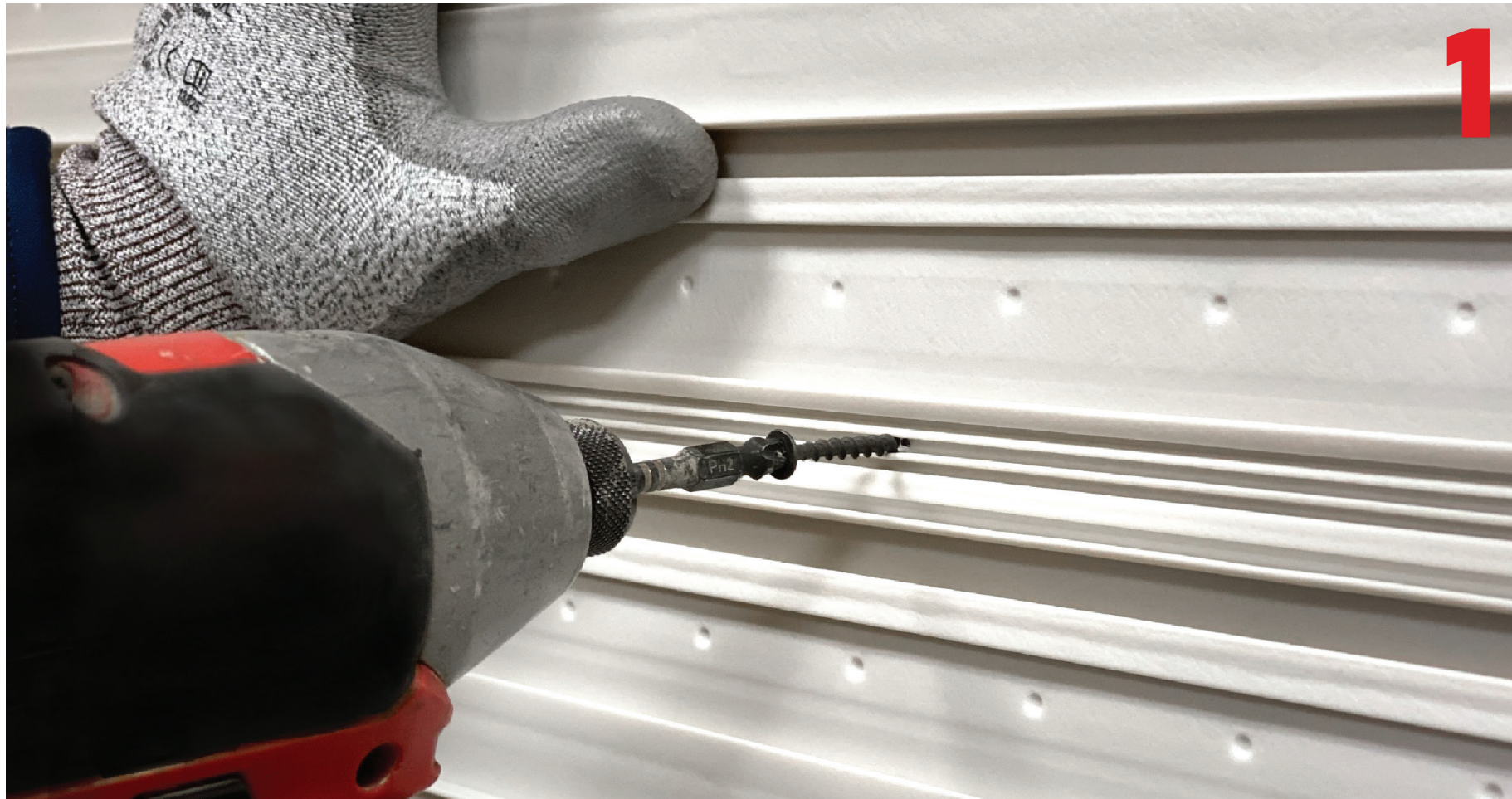
1. Adhere Speedymason Brick Lath panel to surface.
