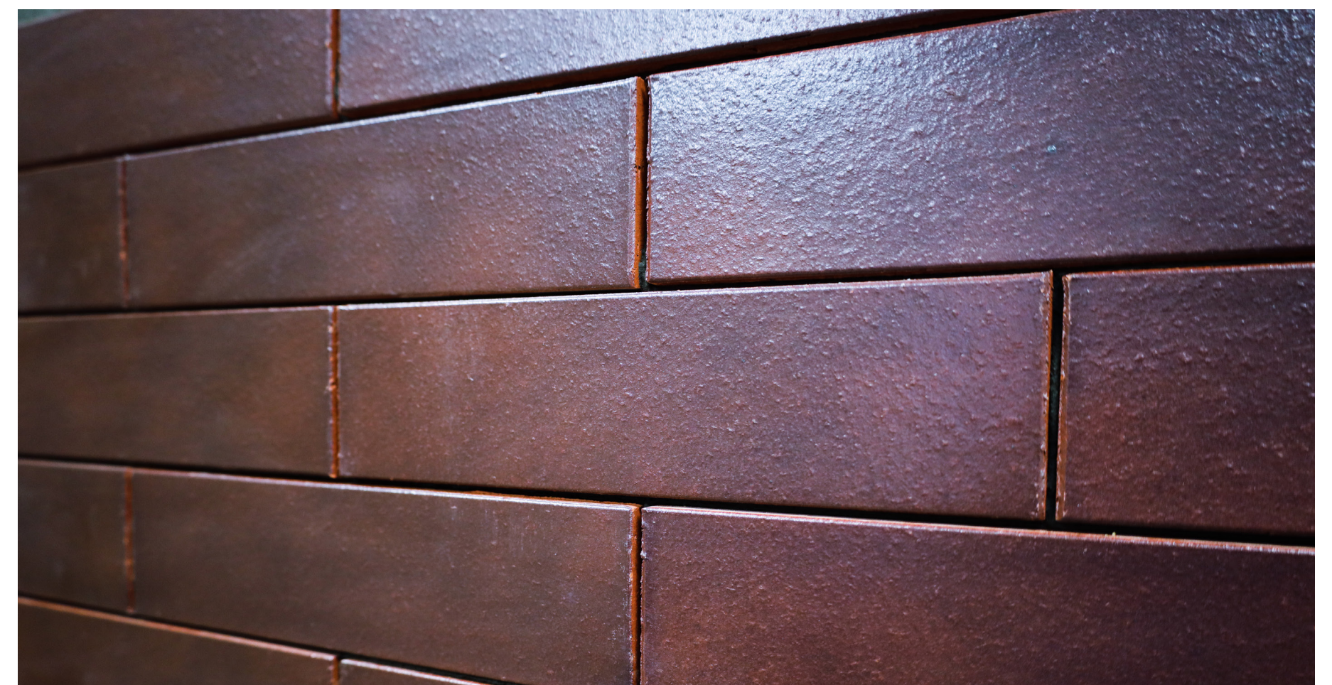
Finished wall with Ultra-Speed thin brick
